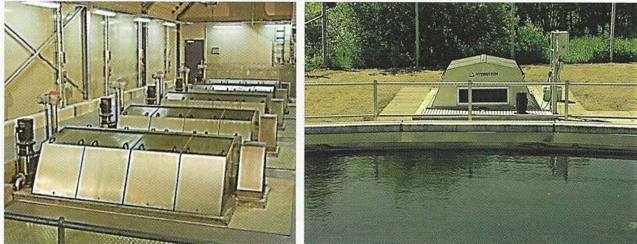
Picture show Hydrotech Discfilters in municipal wastewater treatment plants for effluent polishing. The Hydrotech Discfilter is also used for filtration of intake water to municipal and industrial water supply systems, process water and effluent from pulp and paper industries, food industries, aqua cultures systems and many other applications.
